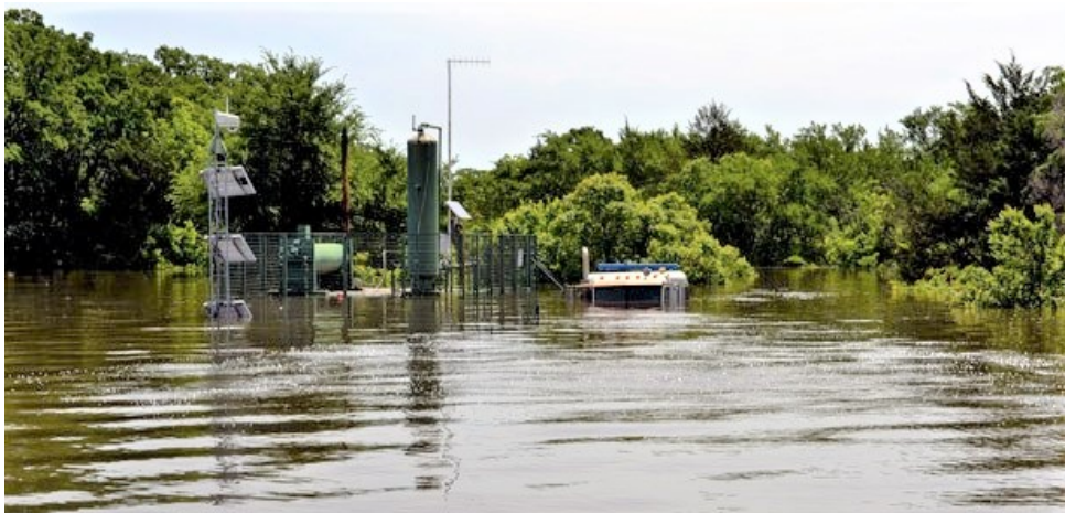
Natural Gas Well Submerged by Lake Texoma Flood Waters 2015
